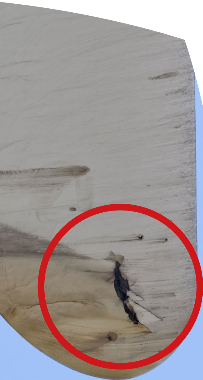
HD blade inspection close-up
